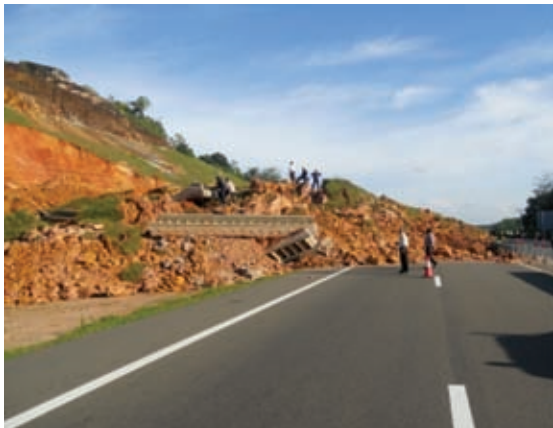
Fig. 11.18 ▲ An occasion of a landslide
