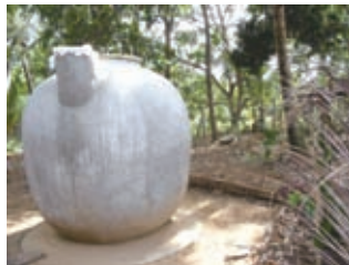
Figure 9.16 - Rain water tanks
