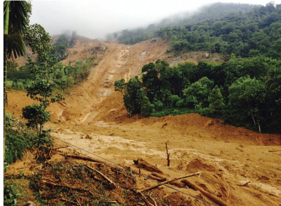
Figure 15.8 ▲ A location of landslide
