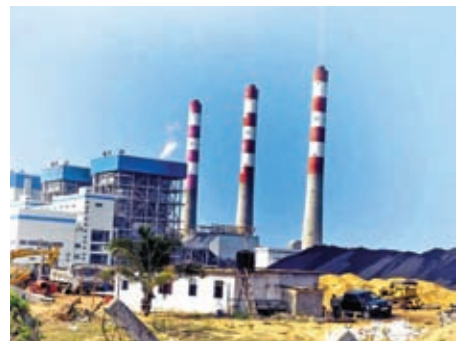
Norochole power station
