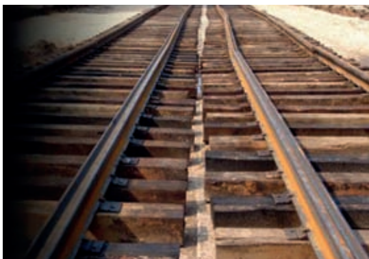
Figure 19.15 (a) – Sleepers on railway line
