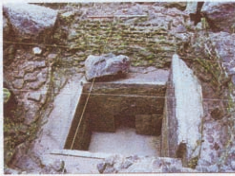
Figure 15.40 - A sluice gate
