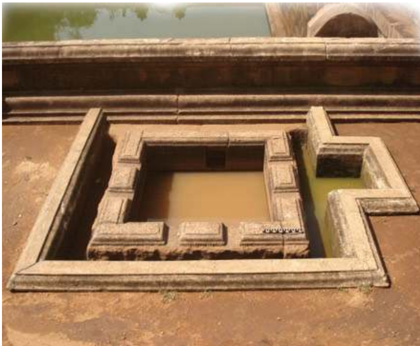
Fig:1.12 A water filter of the Twin Ponds (The water that gets collected in the outer compartment of this filter flows into the inner compartment over the six cuts on the top of the middle wall. Then the water flows from the inner compartment into the pond through a pipe.)
