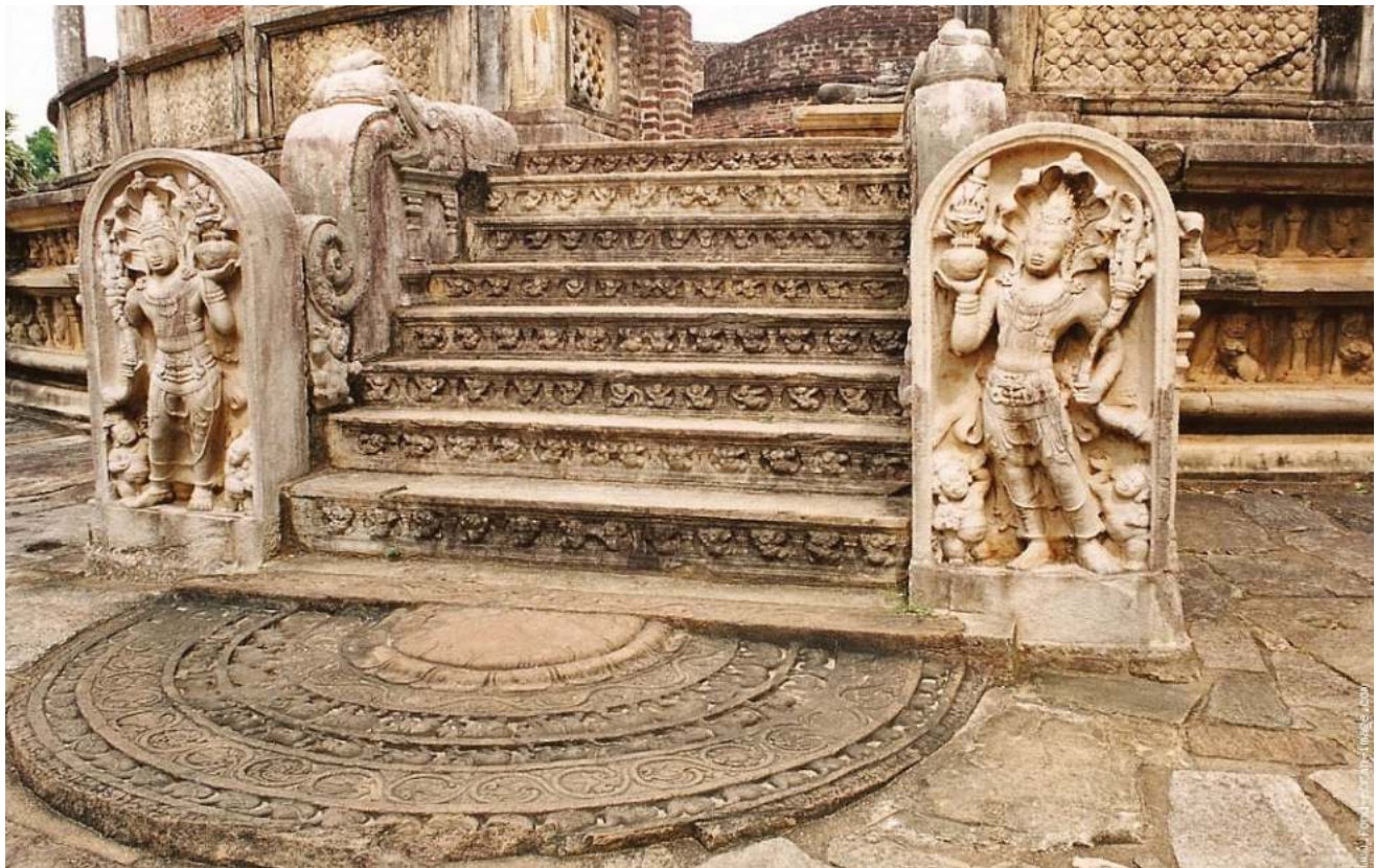
Fig. 1.31 How the Sandakadapahana, guard stones, and Korawakgala had been fixed at the entrance to a building.
