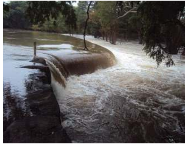
Fig:1.7 Thekkam anicut that has been constructed by building up a dam on a natural rock plain in Malwathu Oya (on the left) and how the anicut overflows after it has been filled with water (on the right).
