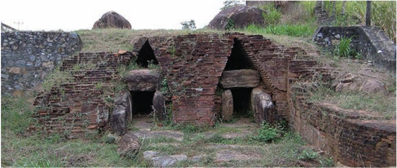
Fig. 5.1 In the place where foreign engineers recommended to construct the sluice gate of the present day Maduru Oya dam, a sluice gate which had been built hundreds years ago, was discovered. These are the ruins of that sluice gate.
