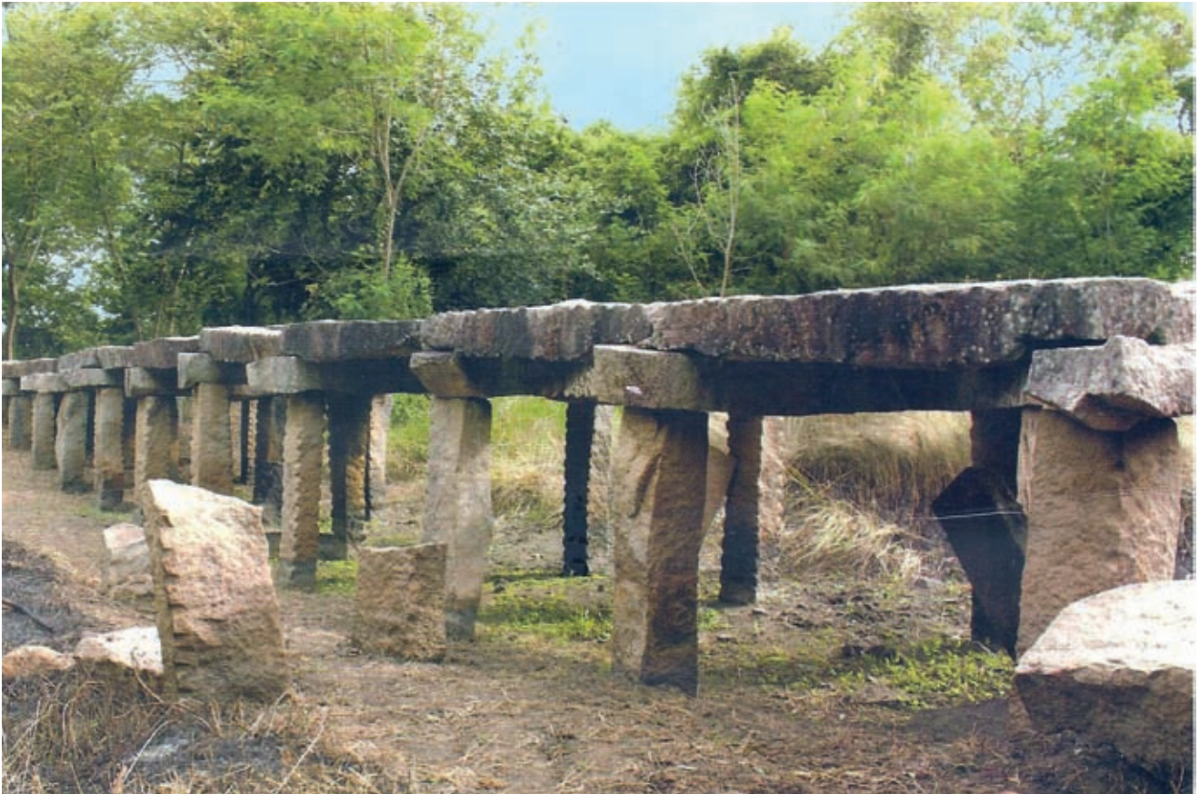
Fig. 5.2. There was a road system stretching from Anuradhapura at that time. The road engineers of that time built bridges out of granites to cross the Malvathu Oya flowing across Anuradhapura. It clearly shows that they had known the basic scientific theory of constructing bridges. These are the present ruins of a stone bridge built so.
